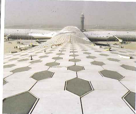
Above right Textured canopy underbelly Right Hexagonal skylights on the back of one of the linear volumes Next spread Undulating honeycomb roof surface above departures concourse and arrivals below
