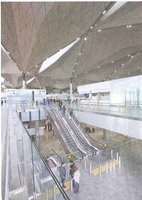
Below Visually connecting the levels, the main floor slab is removed at key points.
