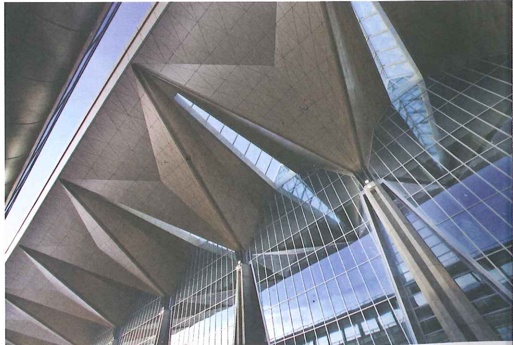
Below A series of rooflights are expressed as sharp cuts in the folded-plate roof.
